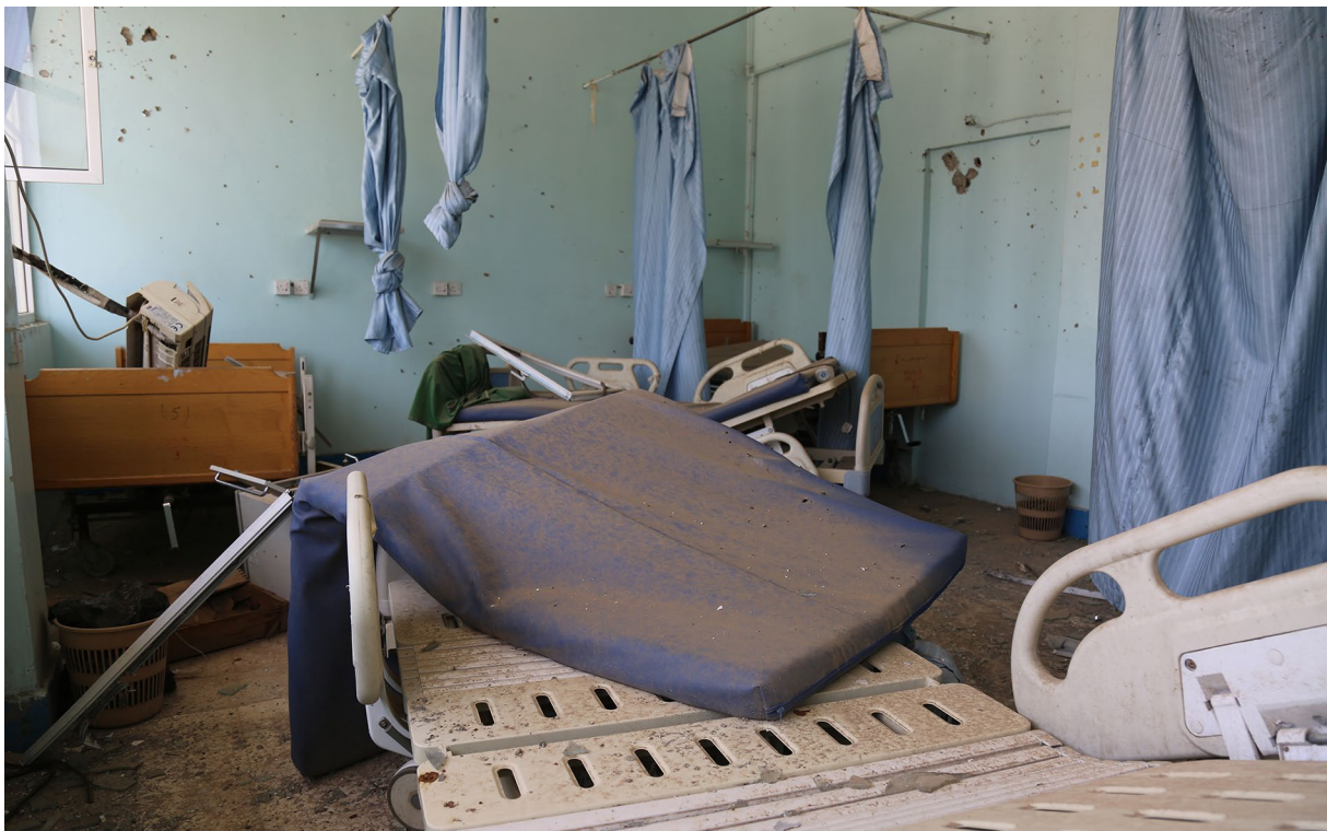
Destruction of Al-Thawra Hospital in Taiz due to shelling by Al-Houthi militia, Shutterstock 1544965799.
